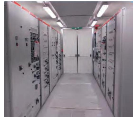
The LER is divided in more modules to allow the shipping and transportation to the site. The LER is placed in site and assembled together to obtain the designed configuration. Each module is manufactured by a structure suitable to be transported and lifted on site with all the internal accessories, cabling system, racks and equipment pre-fitted, excluding batteries to be installed by the installers directly on site to avoid problems during transportation.
